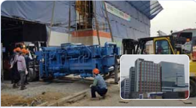
Hwaeom Building Munjeong-dong 2AB 270usRT(949kW)
