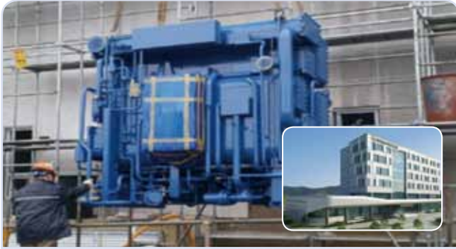
Korea Elevator Safety Agency 2AB 150usRT(527kW)
