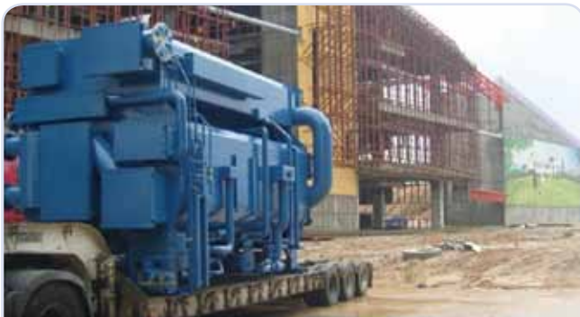
Chungcheongnam-do Provincial Government Administration Building 2AB 2,400 usRT(8,438kW)
