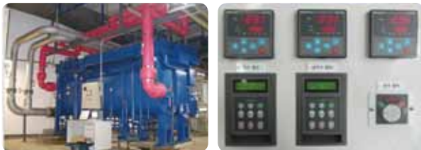
▲ 1st Generation Single Effect Double Lift Hot Water Driven Absorption Chiller
